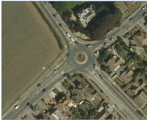
Figure 16 - A256 / A255 Dane Court Roundabout
