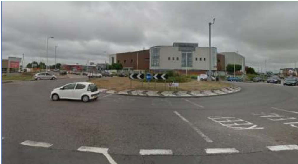
Figure 4 - Westwood Roundabout (A256/A254)
